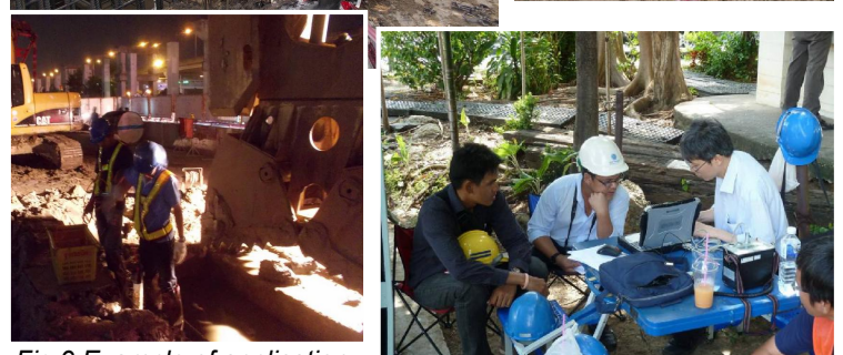
Fig.9 Example of application measure the actual lateral movement of soil near underground tab water tunnel during Barrette pile construction. Measured data of each step are calculate immediately and present on site, continuously 72 hrs.
