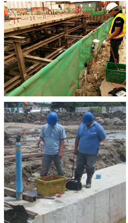
Fig. 4 inclinometer reading on site
